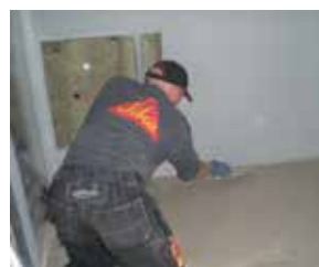
Application of Sikafloor® Marine-100 or -120
