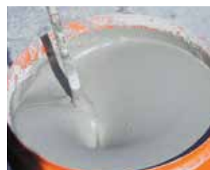
Mixing of Sikafloor® Marine-100 or -120
