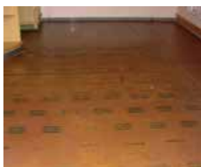
Priming of steel deck with Sikafloor® Marine Primer C
