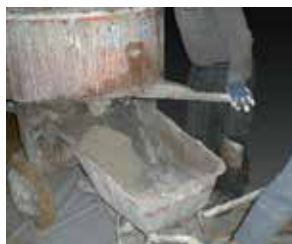
Mixing of Sikafloor® Marine KG-202 N and KG-404 N
