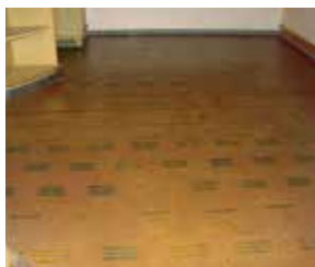
Priming of steel deck with Sikafloor® Marine Primer C
