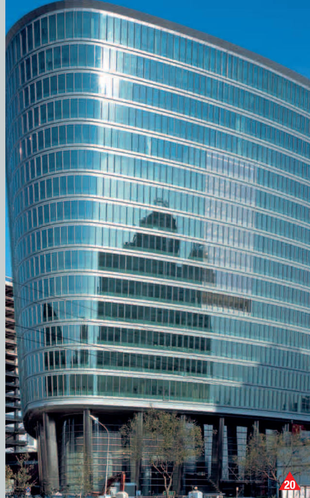
CNOOC Building, Beijing, China; Kohn Pedersen Fox Associates PC
