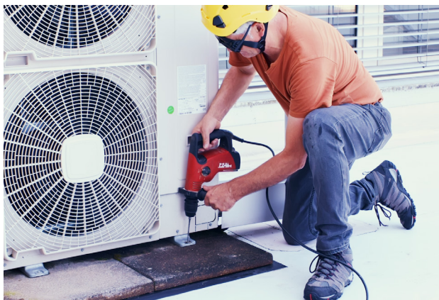
Drilling holes into roof waterproofing membrane by installing various equipment after completed application.
