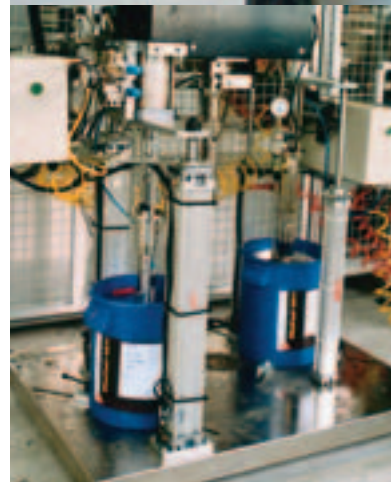
Transfer pumps to feed robot system out of pails
